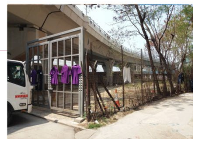
Existing fenced off area
