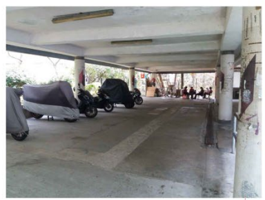
Existing Pier Canopy: To be dressed up
