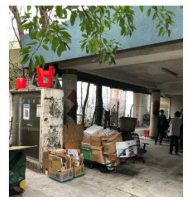
Existing Pillar Box for Public Pier: To be retained at this stage and relocated later
