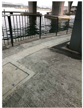
Existing Sloped Walkway: To be modified
