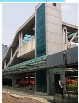
Existing Covered Walkway
