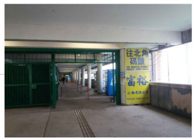
Existing Area under Pier Canopy
